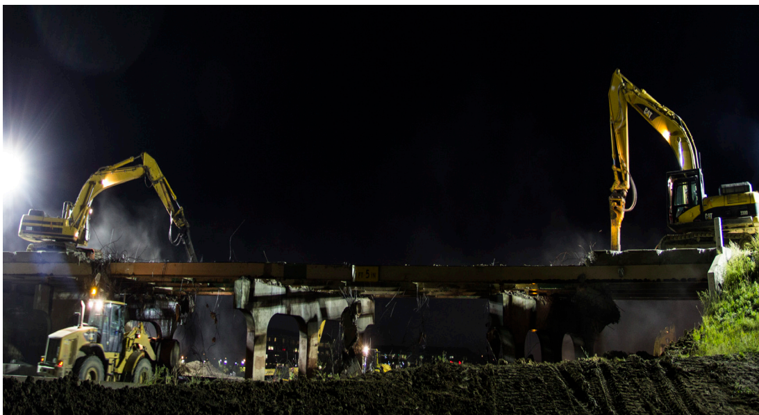
Heavy equipment working in tandem to demolish the Olde Wadsworth bridge.
